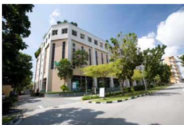
11 Changi South Street 3
